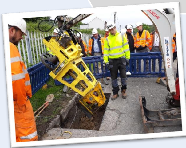
Above: Pipe Puller lowered into place. Right: UPVC pipe being pulled and wound.
