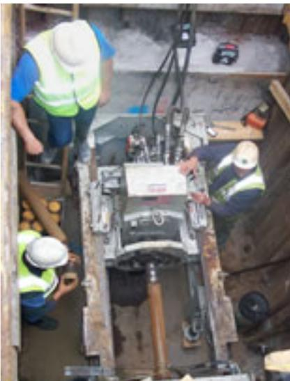
2. Drive pit - Installation of a pilot tube
