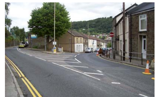
Junction of Park Street / Forest Road
