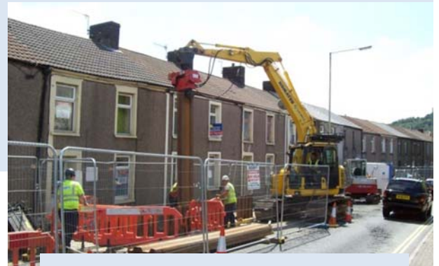
Sheet piling to South connection point.
