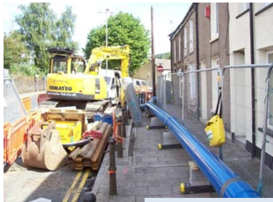
Temporary welded steel overland rider
