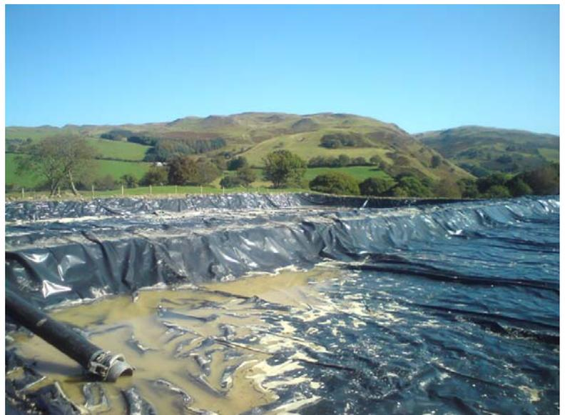
The top lagoon was capable of storing the full capacity of the 400mm pipe. This lagoon would store the dirty water allowing it to settle out the manganese particles before running over a weir into the second lagoon before being released back into the nearby river.
