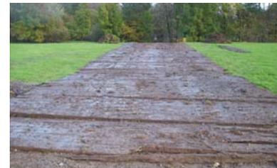
**BA SECTION**—The location of the burst main on the 500mm GRP main was situated in the grounds of the BA site within a lawned area. A bogmat road was constructed over the lawn area to gain access to the burst. The GRP main had ruptured on a 33' bend covered in concrete. All concrete had to be carefully removed from the GRP main without damaging the remaining pipe.
