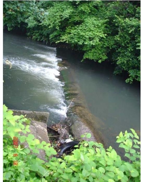
As part of DCWW planned capital maintenance programme LCE were allocated this scheme which involved the removal of an existing 900mm diameter concrete sewer which was acting as a weir across the River Ebbw.
