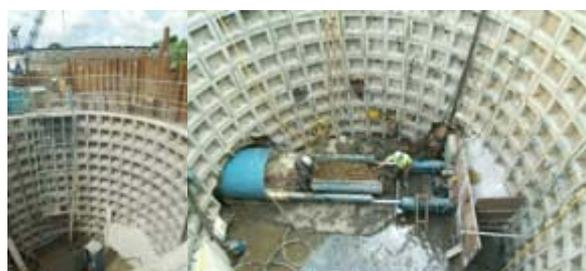
*Tunnelling under the canal from Tank One*
