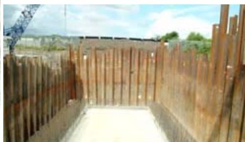
*Overflow tank piled and ready for concrete lining.*
