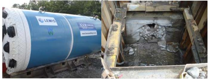
The work was carried out on the Felindre to Margam 43" diameter high pressure steel water main. The main was in poor condition and was leaking significant volumes of potable water. We were informed that the leaking main is sleeved and was safe enough for our work to proceed. The water main remained in operation throughout the course of our work.
