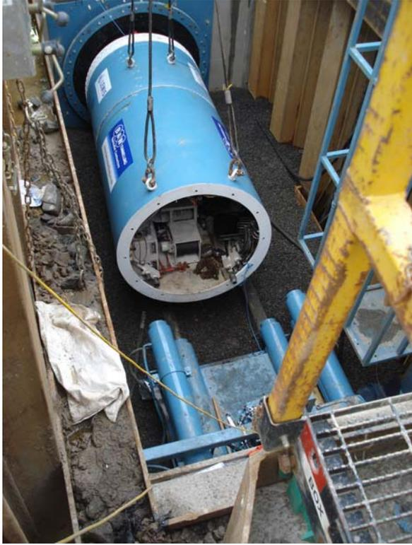
Full Faced Shield Tunnel Boring Machine" (TBM) was used by B&W Tunneling Ltd to bore and pipe jack the 1500mm dia concrete pipes beneath the railway line and Tennant Canal.
