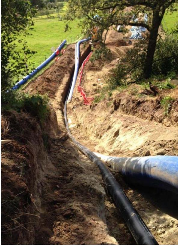
Due to the steep angle, there was a relative risk of slope instability and washout of the backfill material. To ensure stability throughout and post construction, the trench was hand dug and backfilled with bagged granular material, with a geocell grid placed over the entire topsoil stripped area.
