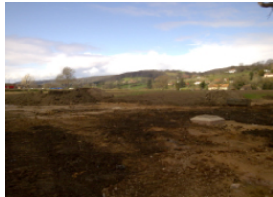
Reinstatement works for the scheme
