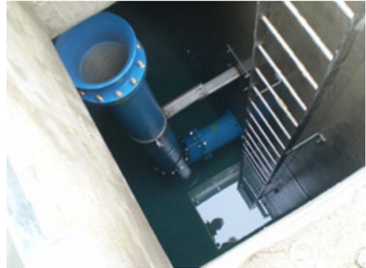
Construction of a 2.5 million litre potable water reservoir & associated pipe work which includes 7 smaller chambers and over 700m of ductile iron pipe and fittings for Wessex Water.
