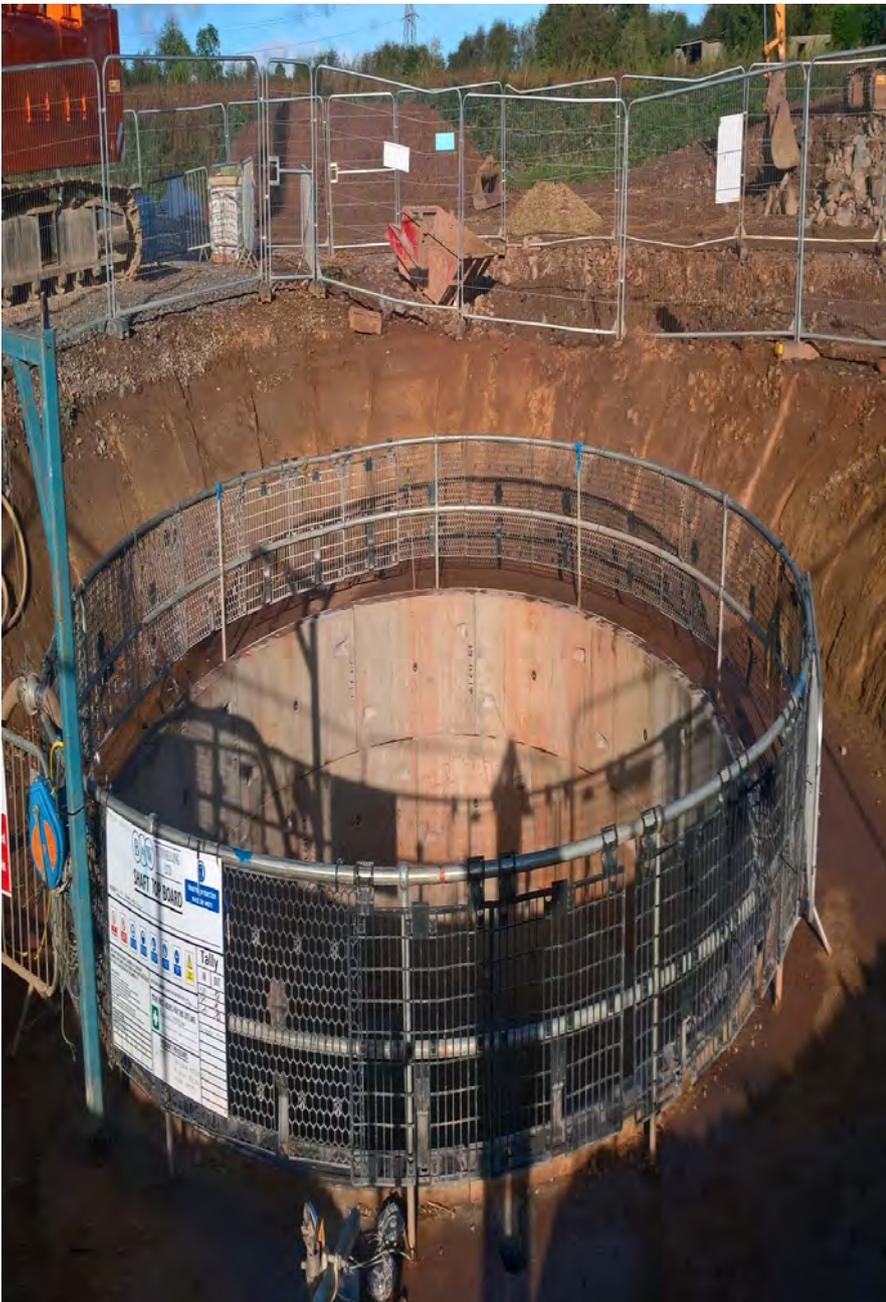
Ground conditions consisted of soft-Mercia Mudstone. And solid rock in places Lewis Civil Engineering development allow the concept of constructing of two segmental shafts structure on a full Design & Build basis.
