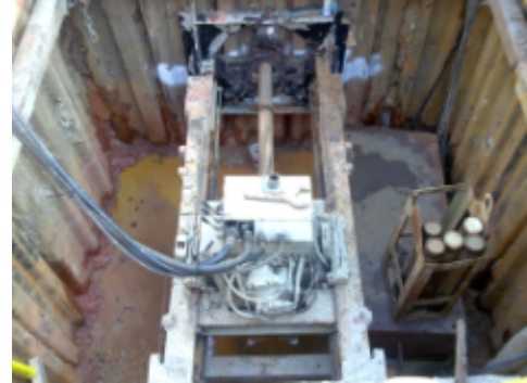
Auger boring process
