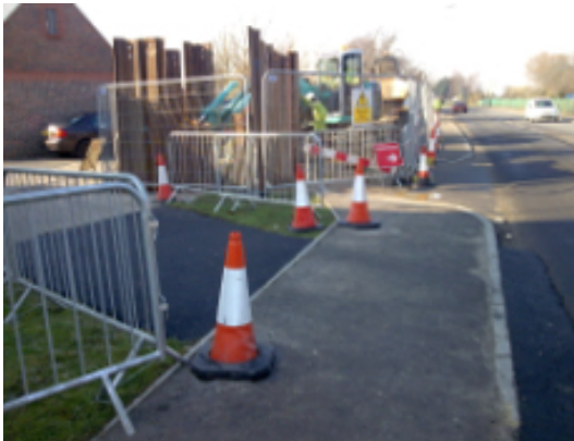
Accommodation works necessary
