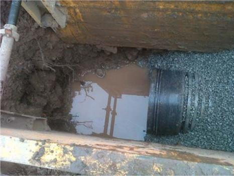
Lewis Civil Engineering Ltd, were engaged by Dwr Cymru under their reactive planned maintenance framework to repair a 600x450mm brick egg storm sewer collapse 3.5m deep within the landscaped grounds of Christ College in Brecon.
