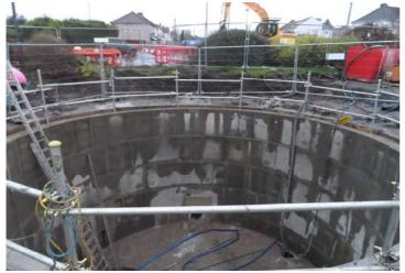
Ground conditions dictated that the shaft was sunk with a cutting ring for the 5m, with the last 2 rings being underpinned.
