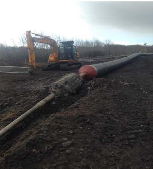
Once the sleeve and the pipe were installed, the annulus between the two pipes was grouted to ensure all voids were filled.
