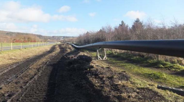
A 100t directional drill rig was used to drill to a set location on the far side of the Railway Line. The 800mm sleeve pipe was then pulled through this pre-reamed hole.
