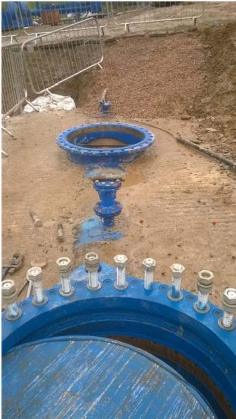
Lewis CE were contracted by Dwr Cymru Welsh Water to replace the 4 butterfly valves within the valve house. This required the excavation of both the inlet and outlet mains and the temporary isolation the flows from both the inlet and outlet mains below the reservoir in a near by field. This would be achieved by installing double flowstops on both mains at the same time.
